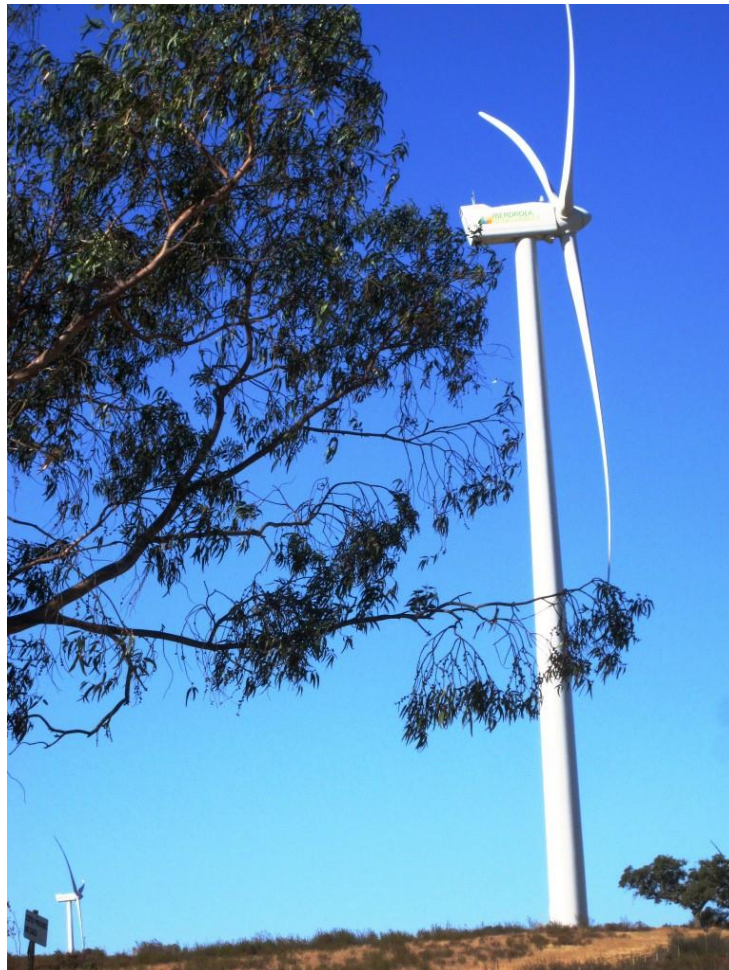
Figure 6.- “Los Lirios” wind farm
