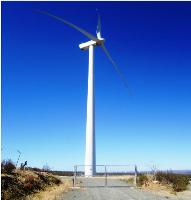
Fig.1 “Los Lirios” Wind Farm
